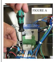
Figure A. Using the screw driver provided, remove the wires that need to be replaced.
