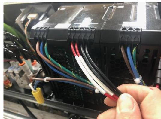
10. Wrap the new wires and existing black wires with the provided black wire sleeve. Make sure that the wires are completely encased.
