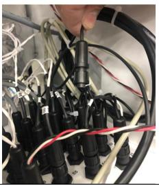
11. Cut the zip tie holding the wires together.
