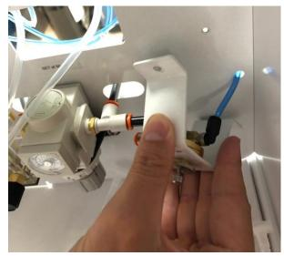
Conduct a pull test the tube to make sure it is properly connected.
