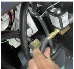
7. On the front right side of the electrical cabinet, move the hose clamp down the hose to loosen and remove.
