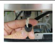
30. Feed the cable through the explosion proof fitting until the black insulation shows through the top about 1". Ensure that the nut tightens on the black insulation so it does not damage the wire itself. Pull the wire gently to make sure it is secure.
