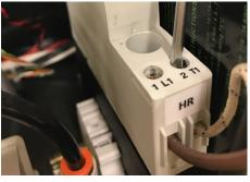
35. Secure the blue cable and both In-Line Heater conductors together with a cable tie. Carefully cut off excess from cable tie without damaging any insulation.
