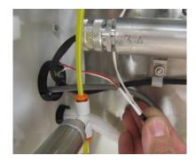
12. On the right side of the Electrical Enclosure, use wire cutters to carefully cut the cable tie that is holding the two white In-Line Heater conductors and the blue cable together, without damaging the insulation.
