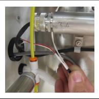
10. Using clippers, carefully cut off both cable ties that are holding the thermistor wire to the two upper brackets of the In-Line Heater. Make sure you do not damage the insulation.
