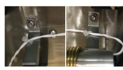
11. Slide out the thermistor from the In-Line Heater. This should easily slide out. If it does not come out, you will need to loosen the threaded plug (Red Arrow).
