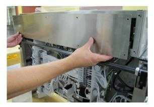
2. Unscrew the 7 screws on the top panel of the electrical enclosure and remove. Set screws and panel aside for reattachment later.
