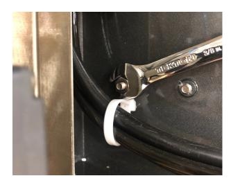
5. Free the cable strap from the back side of the screw.
